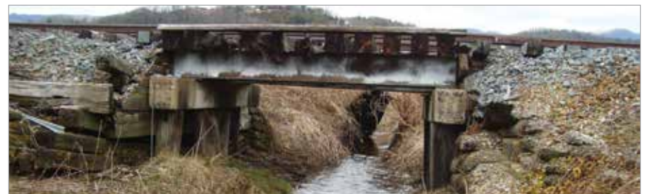
Typical Minor Bridge
